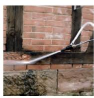
The wet jet unit fits easily on Kärcher high-pressure cleaner spray lances. The abrasive is sucked up, entrained in the water jet and applied with a powerful abrasive action. Ideal for removing rust, scale and paint from components as well as graffiti.
